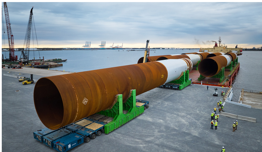
Thus far, 24 monopile foundations have been successfully offloaded and stored at PMT.
