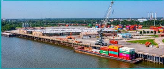
RICHMOND MARINE TERMINAL
